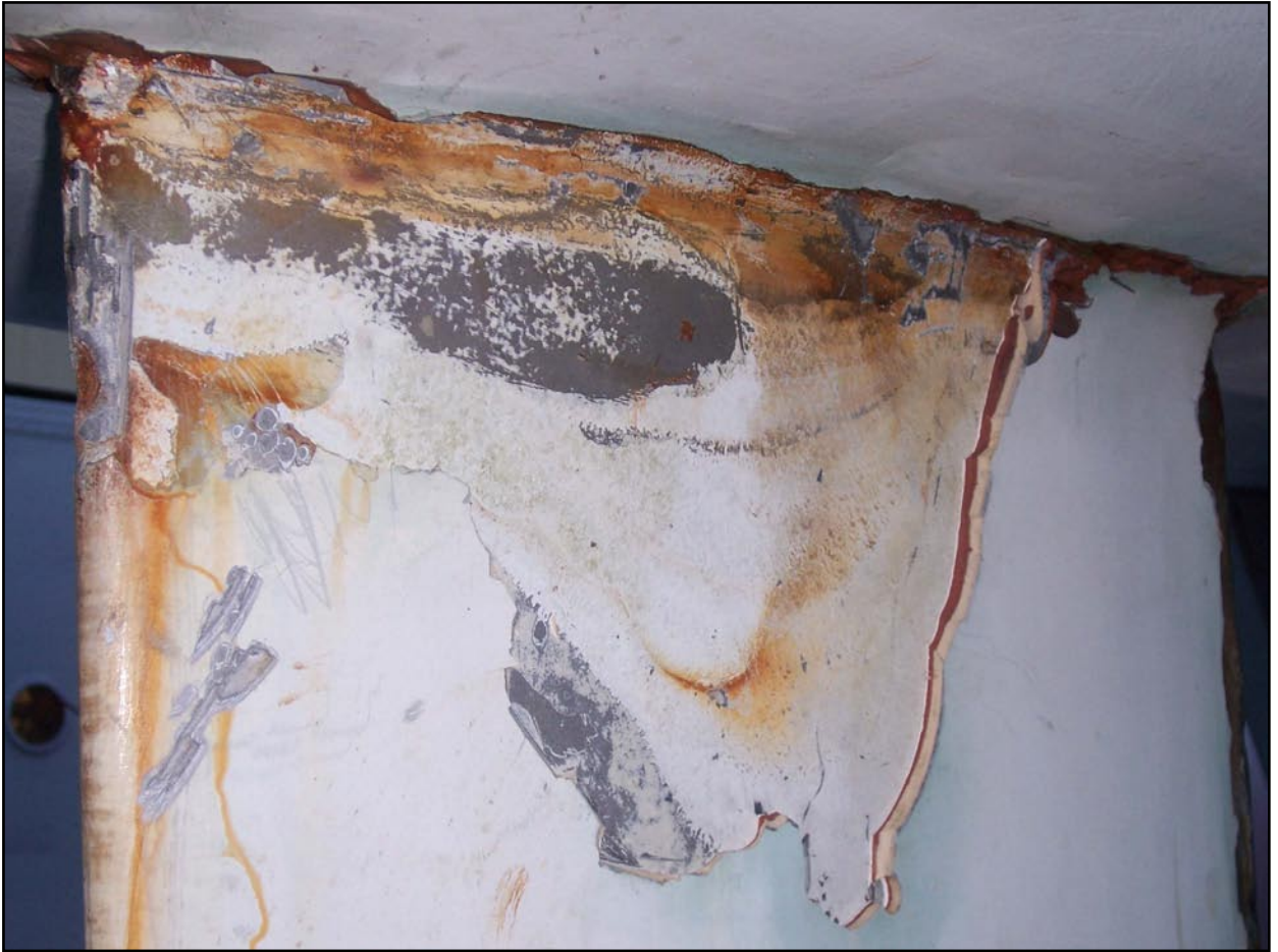
Condition of port side of the keel - November 2006
