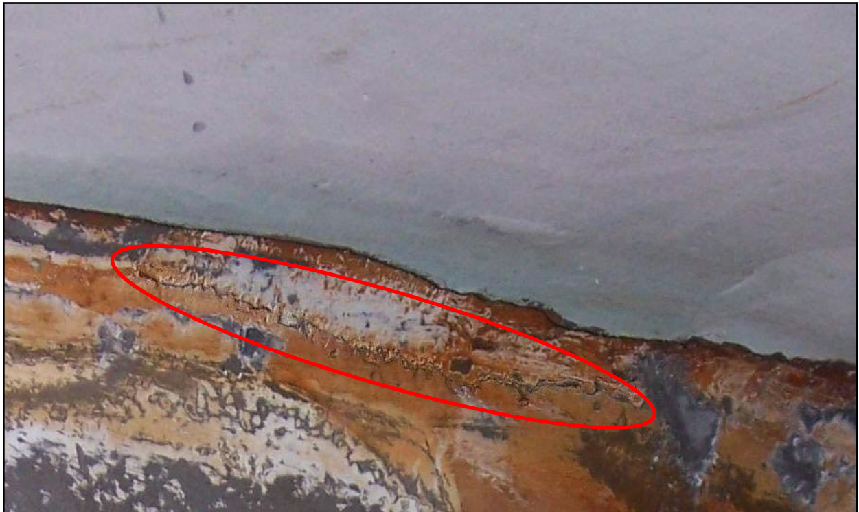
Site of possible crack - port side of keel photographed at Queen Anne's battery, November/December 2006
